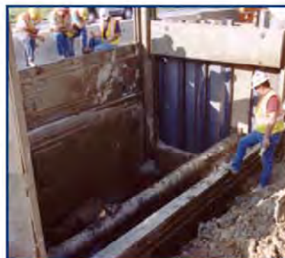
Sheeting Guide Frame/SRS Combo
